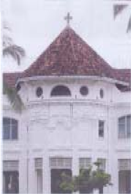
The building at the top of the page is the old school building of the school which was built in 1910 and is now a museum.
